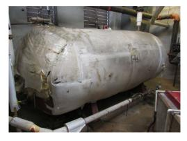
There is really no actual maintenance to the actual storage tank. Check sealed areas, supply and distribution pipes that are threaded into the storage tank for leaks. Any noted leaks should be addressed immediately. The bladder and actaul tank wall thinckness should be tested in order to make sure both are properly working and safe against possible leaking, cracking and major failures.
