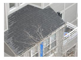
The estimated cost used is for a quality 25-30 year rated asphalt composition shingle, all new underlayment, flashing and drip edge. A provision should be included in any work contract for the replacement of sheathing. Most likely some of the sheathing will require replacement. However, until the roofing system is removed from the roof deck it is next to impossible to know how much if any of the sheathing will require replacement.
