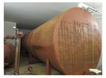
This line item is for the replacement of the main storage tank (25,000gals.), the sub-storage tanks, and the pressure tanks.
