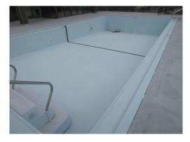
The pool is located on the roof of the building. The pool is a aluminium tub style pool. The
