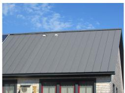
The estimated cost used is for a quality 40 year rated metal standing seam roof system, all new underlayment, flashing and drip edge. A provision should be included in any work contract for the replacement of sheathing. Most likely some of the sheathing will require replacement. However, until the roofing system is removed from the roof deck it is next to impossible to know how much if any of the sheathing will require replacement.
